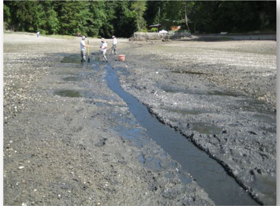
Diverting natural freshwater inputs by digging trenches in an estuary
